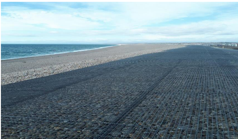
Chesil Beach showing the gabion tower mattress.
